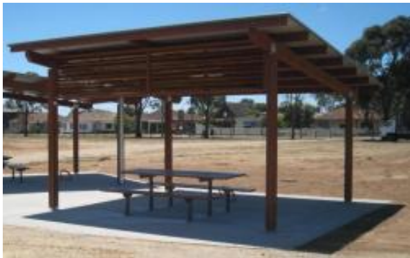
Timber-slat pergola (no roof sheeting)
