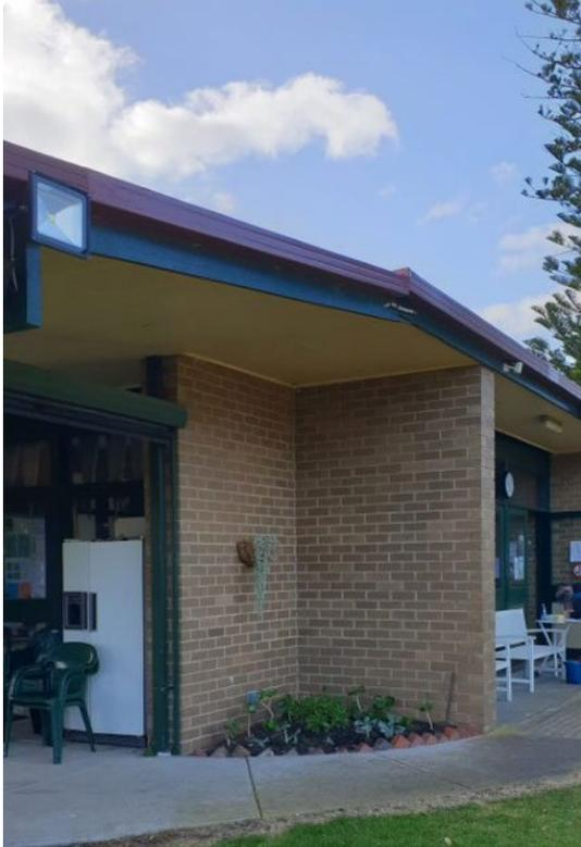
**Figure 5.** Photograph showing the deep eave overhang in 2020 (Source: Context)
