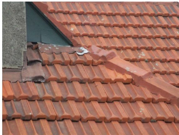
16: Exterior - misaligned flashing and tiles
