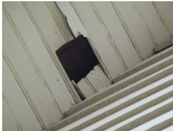
14: Exterior - hole in eaves
