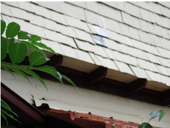
15: Exterior - misaligned flashing and shingles
