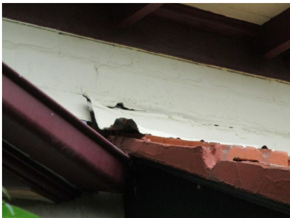
17: Exterior - misaligned flashing
