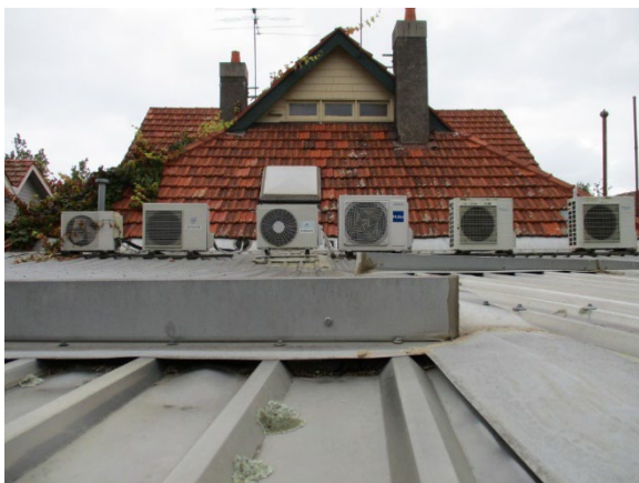
21: Exterior - profile metal sheet extension (2)
