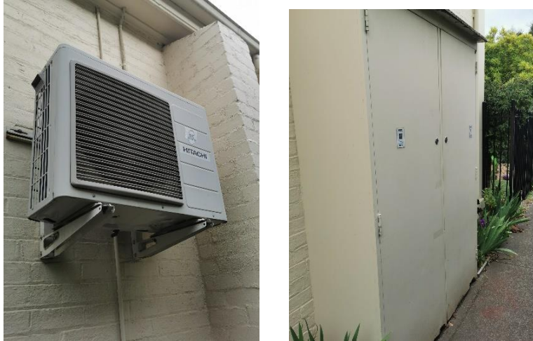
FRONT ENTRANCE SPLIT SYSTEM AND SWITCHBOARD CUPBOARD
