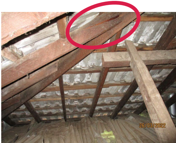
29: Roof Space (3) Cracked Rafter
