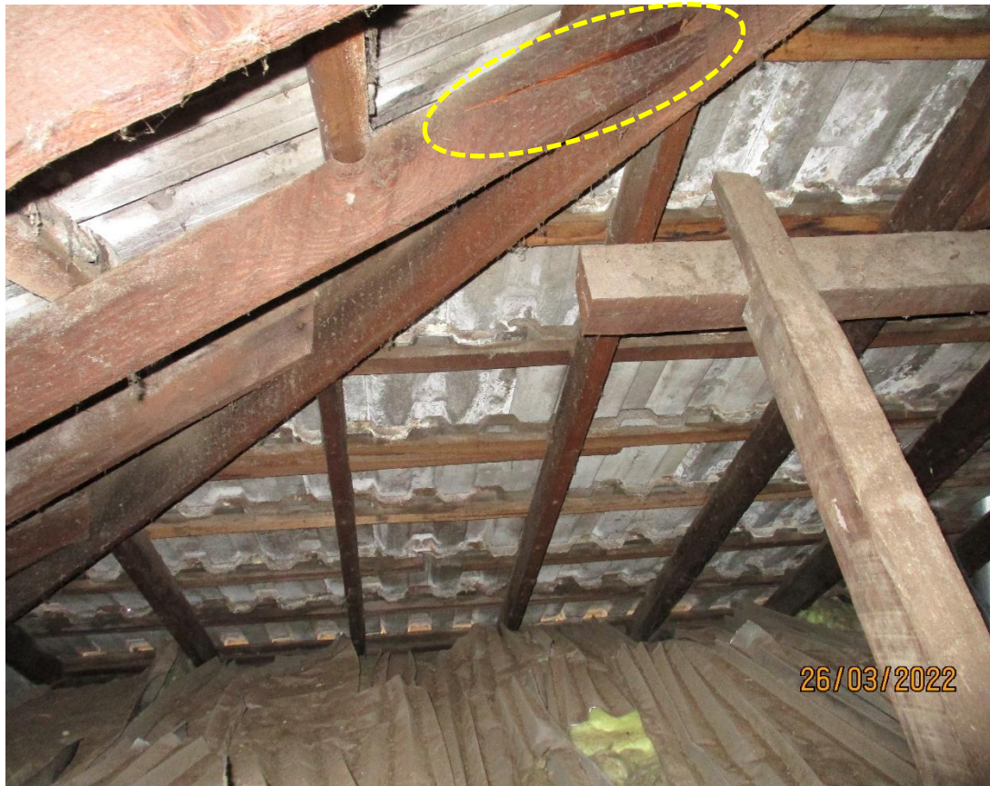
Figure 1. Photograph 29 excerpted from the RZ Report, indicates a split in a timber rafter no.1.
