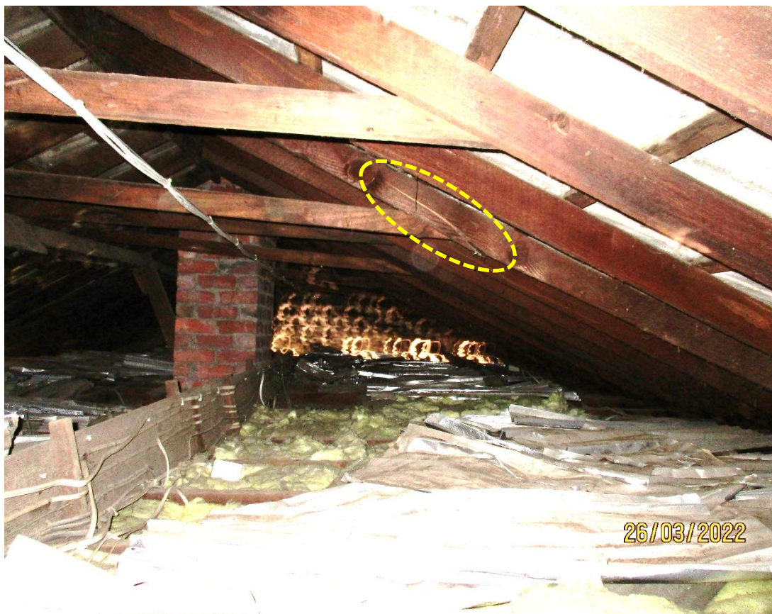
Figure 2. Photograph 30 excerpted from the RZ Report, indicates a split in a timber rafter no.2.
