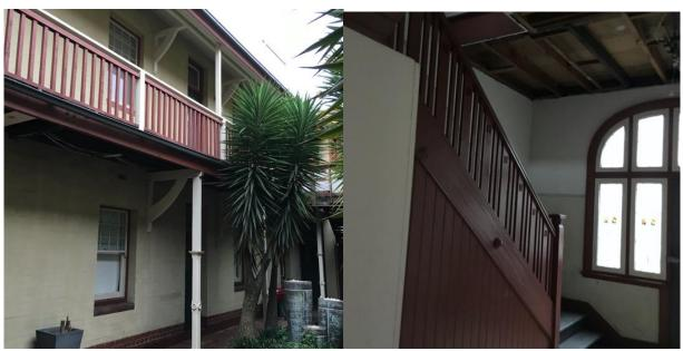
At left shows the external access galleries to the first floor flat facing the internal courtyard — note the original timber bracket (adjoining post is a later addition). At right shows the staircase inside the entrance hall.
