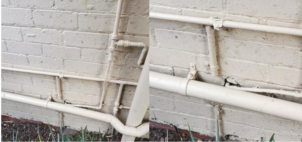
MINOR CRACKING BRICKWORK
