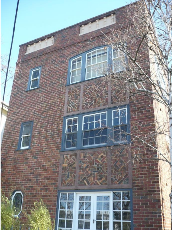
At left: Main elevation of the south block showing panels with brick 'nogging' between the window bays, the Tudor arch to the top window and the inset balustrade panels to the parapet. Note octagonal window lower left (see 'Building details' below)
