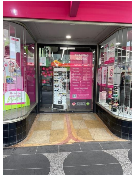
Original shopfronts to Acland, showing (at right) terrazzo floor to the ingos (covered by mat in left image)
