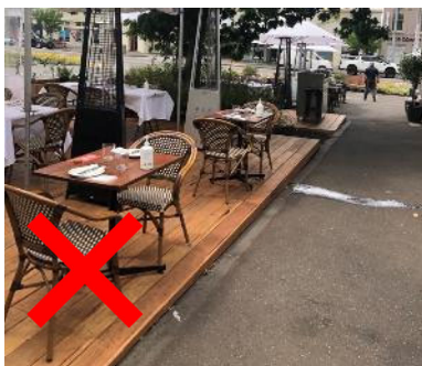
Figure 23: Platform is not flush with surround footpaths.
