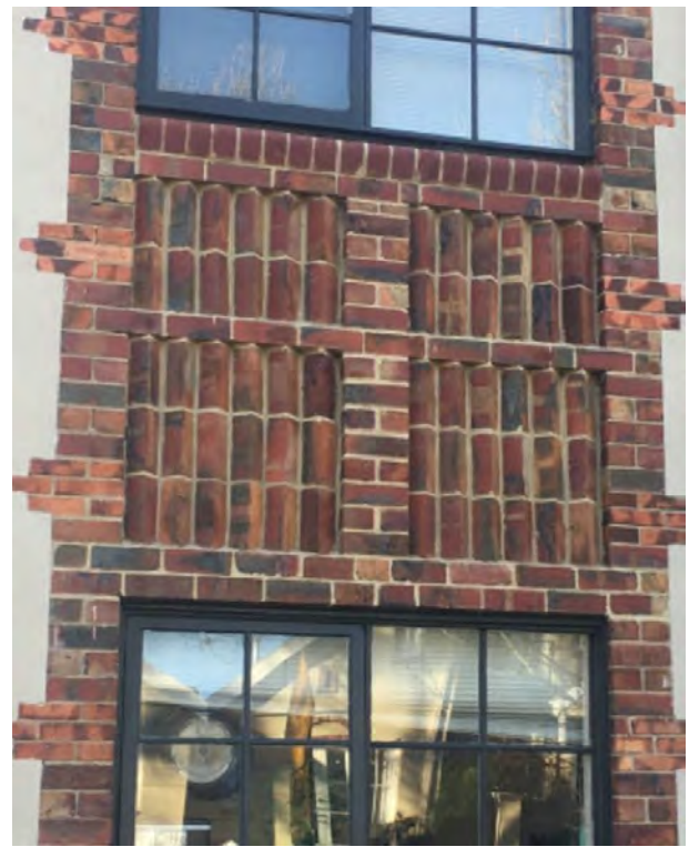
Figure 10. Detail view of sections of angled soldier course.
