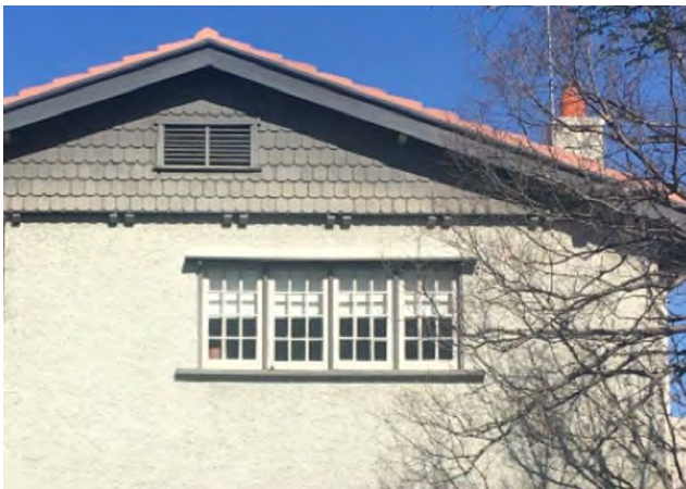
Figure 9. Detail view of shingled gables and grouped casement windows along two-storey gable projection.
