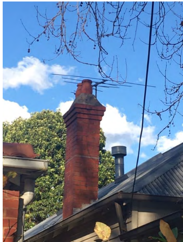
Figure 8. Detail view of face brick profiled chimney with chimney pots.
