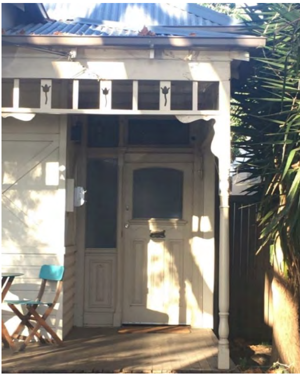
Figure 9. Detail view of turned timber posts, verandah fretwork and entrance door.
