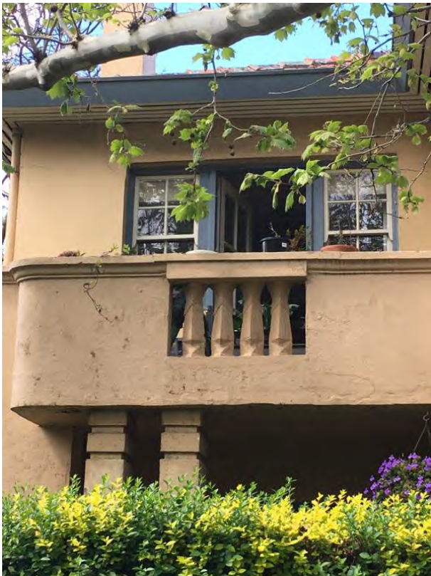
Figure 8. Overview of façade balcony and balustrade with distinctive 'Dorney' balusters
