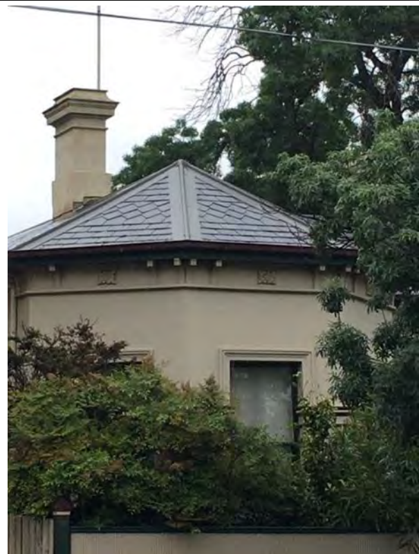
Figure 17. Detail view of the front bay of No. 9 Scott Street showing chimney and diamond slate pattern.
