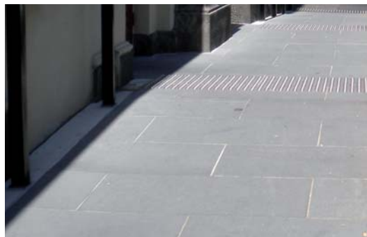
Paving to be sawn bluestone
