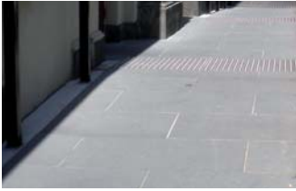
Paving to be sawn bluestone
