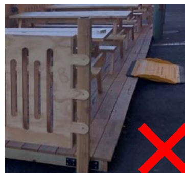
Figure 22: The platform has been constructed at the level of the footpath.
