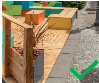
Figure 22: The platform has been constructed at the level of the footpath.
