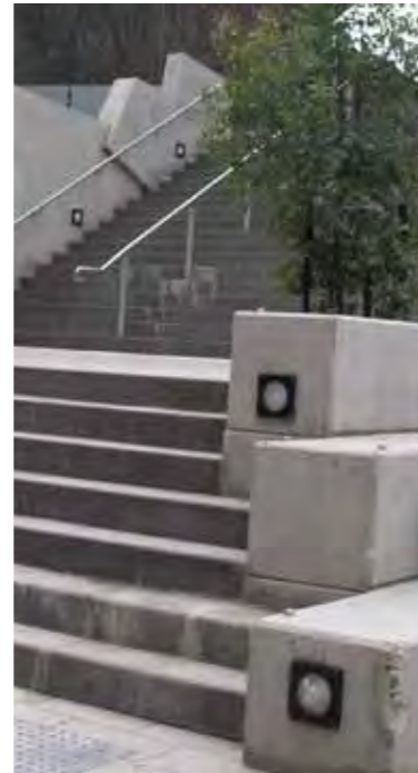
Above: an example of lamps integrated into stair elements
