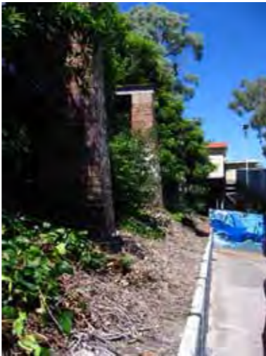
The existing brick platform supports should be incorporated into the new station upgrade
